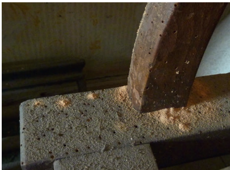
Figure 3.1 Piles of furniture beetle ( Anobium punctatum ) frass.
